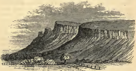
FIG. 51.—View of part of the cliffs and landslide of Antrim.
